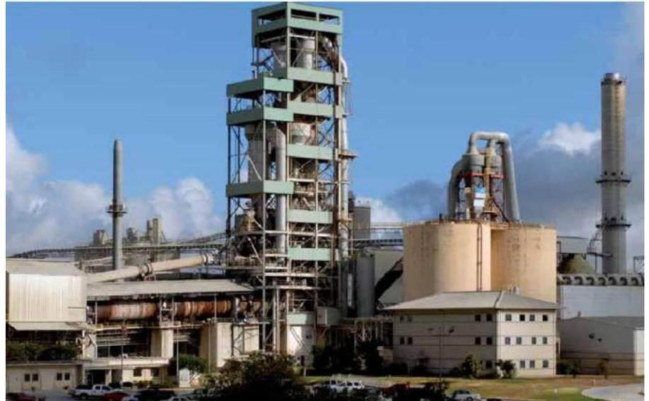
channel Analysis of Soil Waves (MASW) tests on different locations of the Capitol cement plant to accurately evaluate the dynamic properties of the soils. This method is based on the analysis of geometrical dispersion of the surface waves, from the evaluation of the vertical distribution of the dynamic shear modulus of soils. As final result it provides the Shear Wave Velocity profile along the subsoils affected by the wave propagation. SAXUM has extended experience
